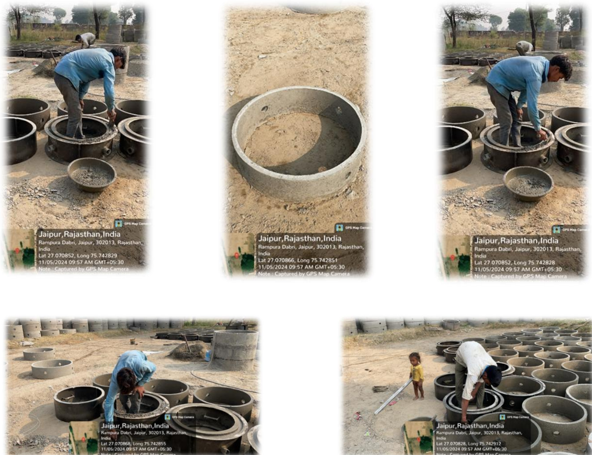
Figure 4: On-Site Assessment of Artificial Reef Deployment: Structural Framework and Installation Process (Source: Captured by Vikas Kumar Ujjania, Author of Book Chapter )
