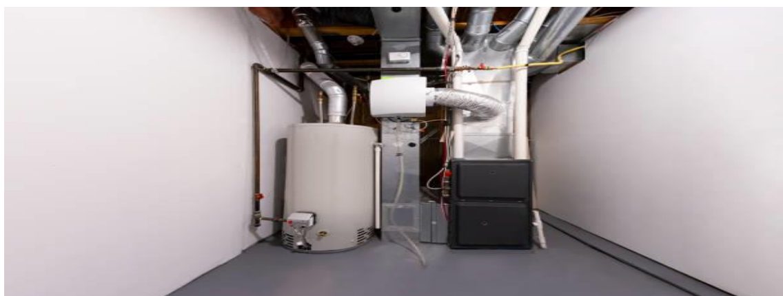
Figure 1: Humidity control system
