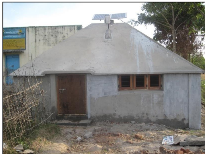
Figure 2: SPR test house
