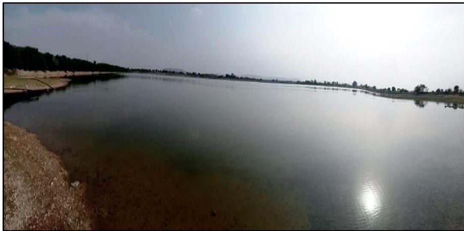
Figure 2: The Gangoti Dam at Gangoti in Tal. Man, Dist. Satara
